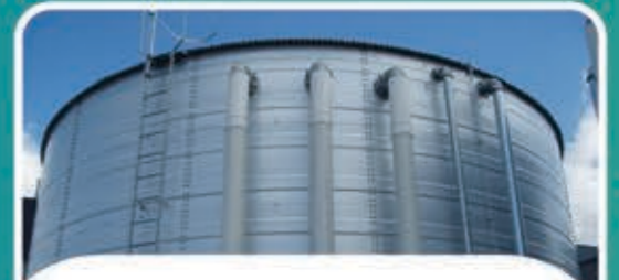
SUPPLY & CONSTRUCTION OF WATER TANKS
