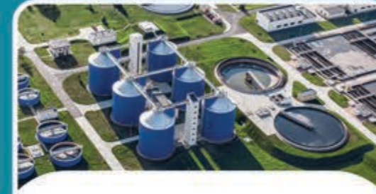
SEWAGE TREATMENT PLANT
