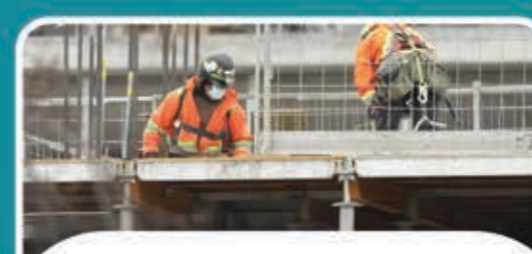
CONSTRUCTION OF REQUIRED BUILDING AT WELL SITE
