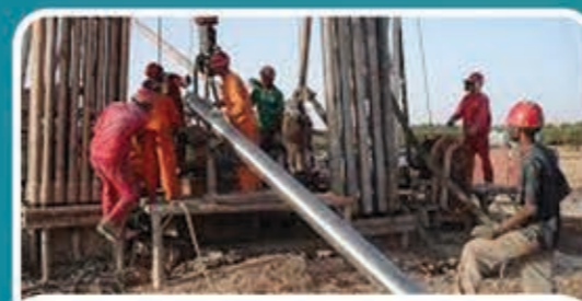
INSTALLING OF CASING & SCREEN PIPES
